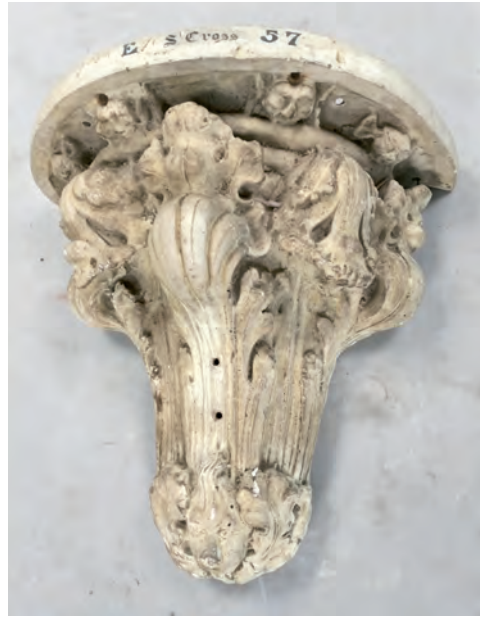
Fig. 3. Cast of bracket (?Early English) from St Cross, Winchester showing heavy undercutting (OAS-E57/OMS-1975.238.84).
