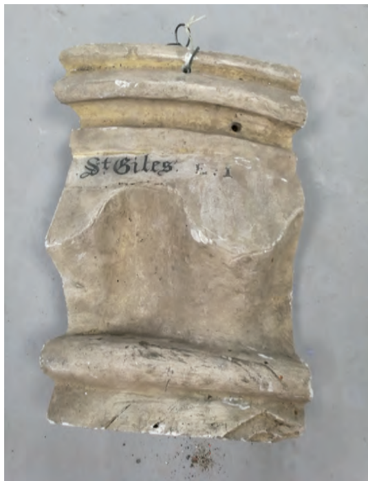
Fig. 17. Section of capital in St Giles' church with 'traces of the cushion form of the preceding period', c.1200 (OAS-E1/OMS-1975.238.28).
