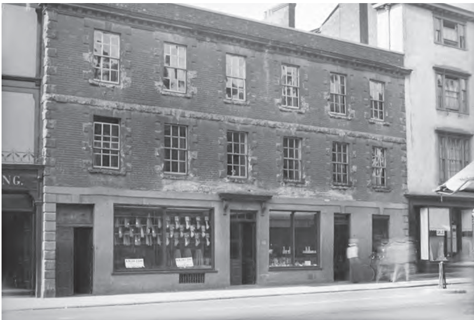
Fig. 8. Nos. 69–70 High Street photographed by Michael Bunney in about 1931, 'before spoliation'. The brick façade with stone dressings was rendered and re-windowed in 1932. HE, BUN01/01/093. By permission of Historic England Archive.
