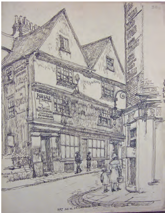
Fig. 7. Drawing by Maresco Pearce showing Nos. 30–28 George Street in 1932. This seventeenth-century house, the last example in the street, was demolished in 1935. Bodl. MS Top. Oxon. b.250, f. 20r. Image courtesy of The Bodleian Libraries, University of Oxford.
