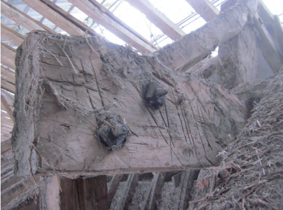
Fig. 18. Baltic timber marks at truss IV (rafter N27). Photo by David Clark.
