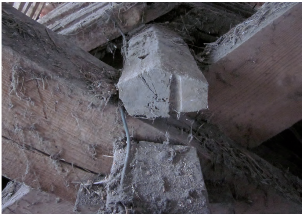
Fig. 14. Truss V – crown plate in foreground. Photo by David Clark.
