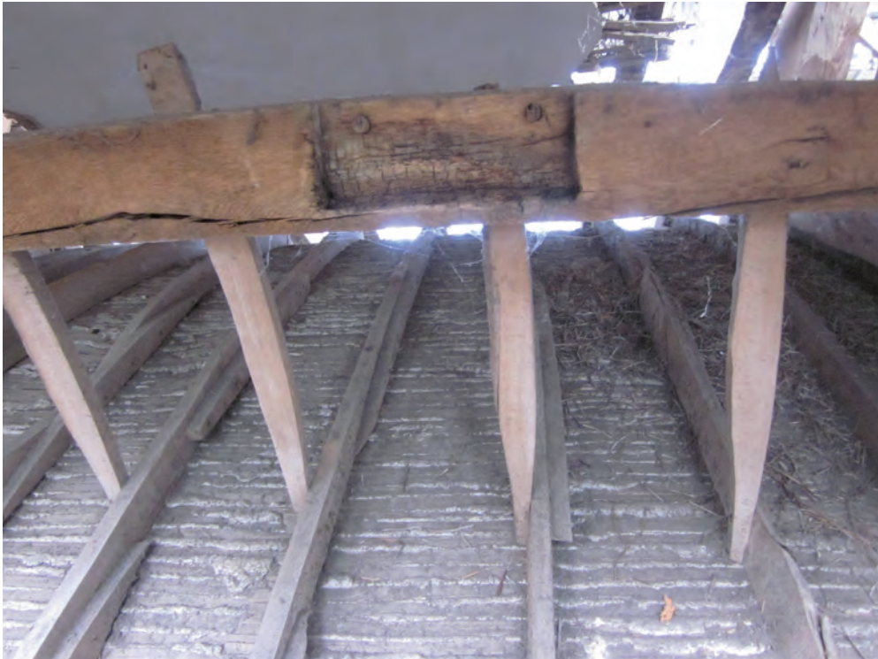
Fig. 19. Purlin in Bay 2 south with struts supporting the ribs of the plaster vault below. Photo by David Clark.
