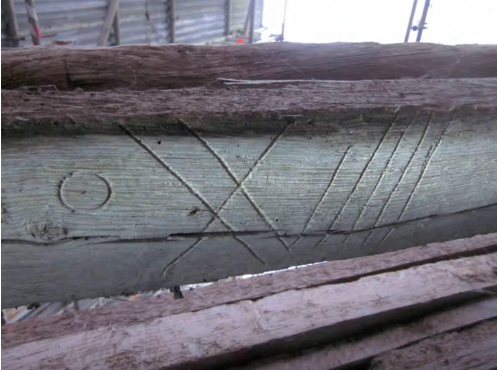
Fig. 16. Assembly mark on rafter S39. Photo by David Clark.
