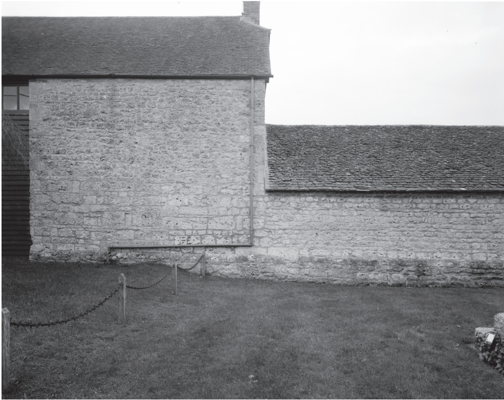
Fig. 3. The north wall of the barn at the extreme west end of the existing building. The westward continuation of the medieval plinth beyond the existing gable can be clearly seen. The vertical straight joint (below the existing gable) marks the corner of the building as reduced in length in the seventeenth century (Period II). The building to the right was built against it, and on top of the surviving medieval plinth, at a later date (Period III). In 1810–11 (Period IV) the side wall and part of the seventeenth-century gable was heightened, creating the building in its existing form. Photograph by Peter Hamilton.
