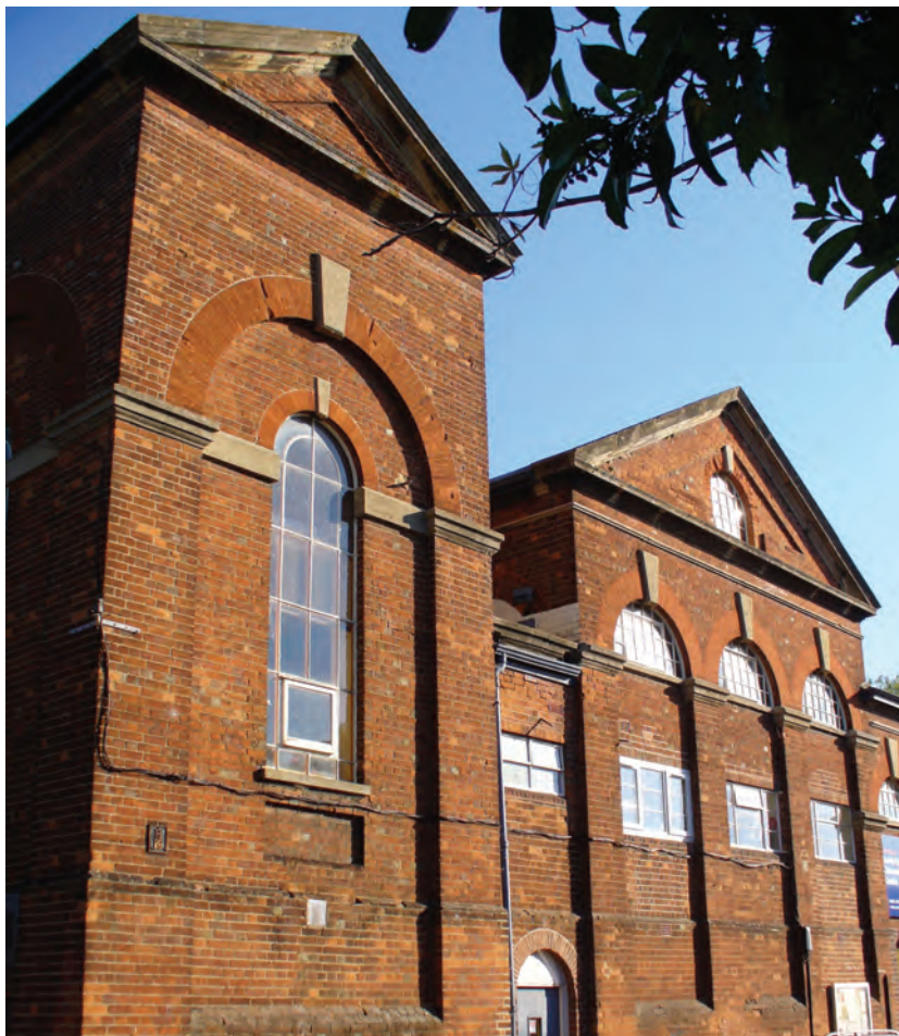
Plate 5. Part of the southern façade of the pumping station at Lake Street waterworks, Oxford, showing the typical high, round-headed windows. The original engine house, on the right, was built in 1856; the Butterly rotative engine house, on the left, was added in 1862. Photograph by author. [Woolley, p. 77]
