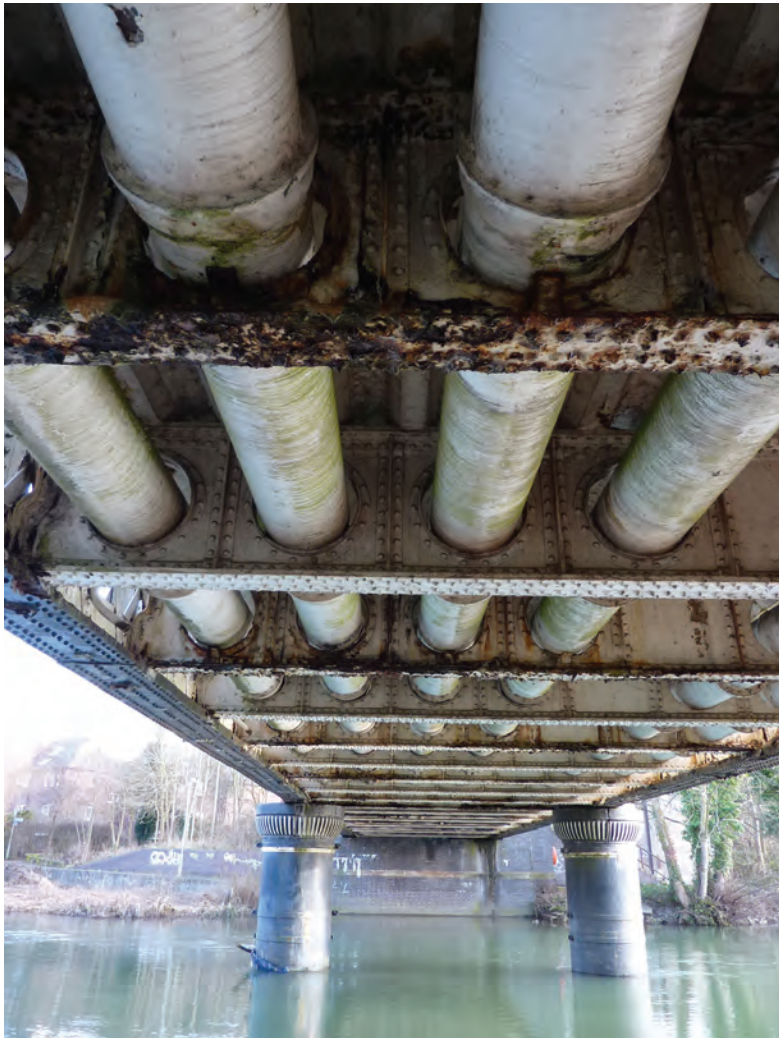
Plate 4. The underside of the St Ebbe's gasworks railway bridge as it is today, showing the two central supporting piers and the mains pipes suspended beneath the floor. Photograph by author. [Woolley, p. 71]
