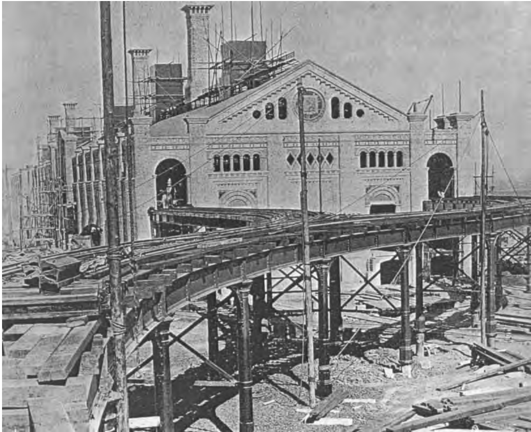
Fig. 2. Retort house designed by F.J. Evans at Beckton gasworks, Woolwich (1869–70), with the railway viaduct to transport coal from the Thames: Edgar Jones, Industrial Architecture in Britain, 1750–1939 (London, 1985), p. 133. Reproduced by permission of National Grid.
