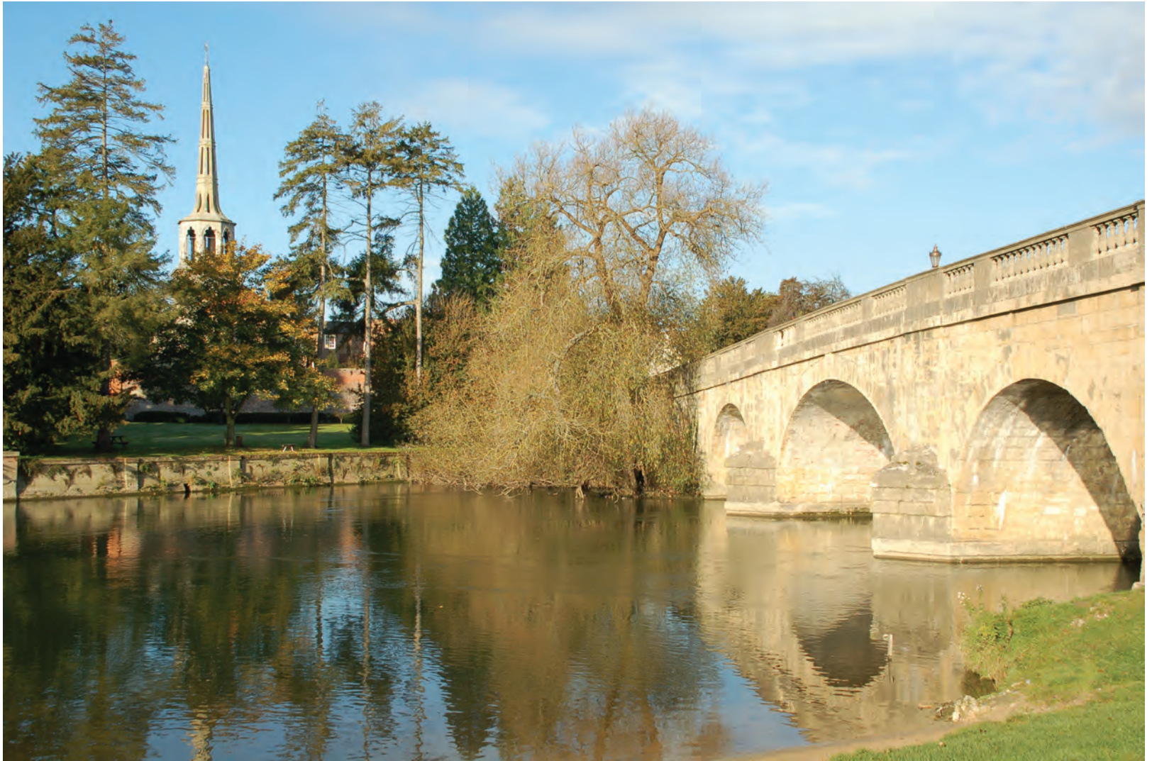
Plate 2. View looking west across the Thames: the spire of St Michael's Church is to the left (this a post-Civil War rebuild), and Wallingford bridge to the right. Only part of the bridge stands in the river itself; the stonework reveals multiple phases of building and repair. [Christie, p. 43]
