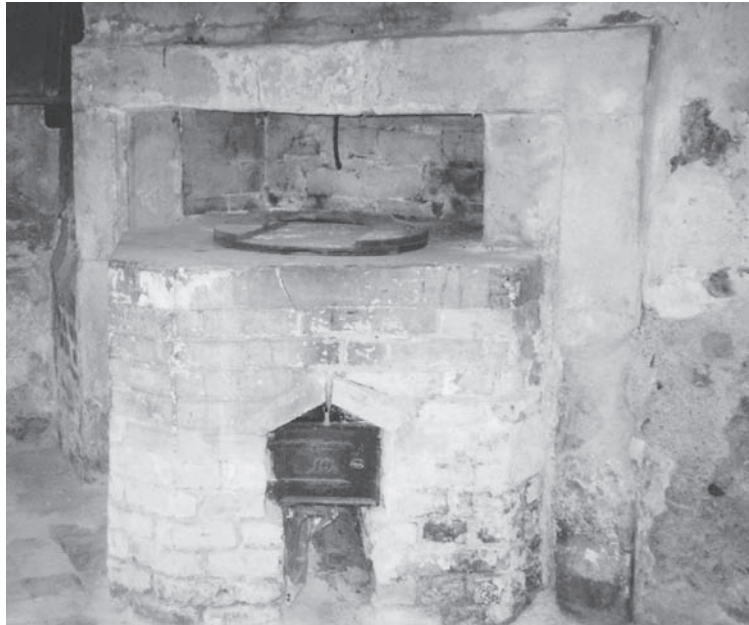
Fig. 5. The copper used for heating water in the basement. ( Photograph by author. )
