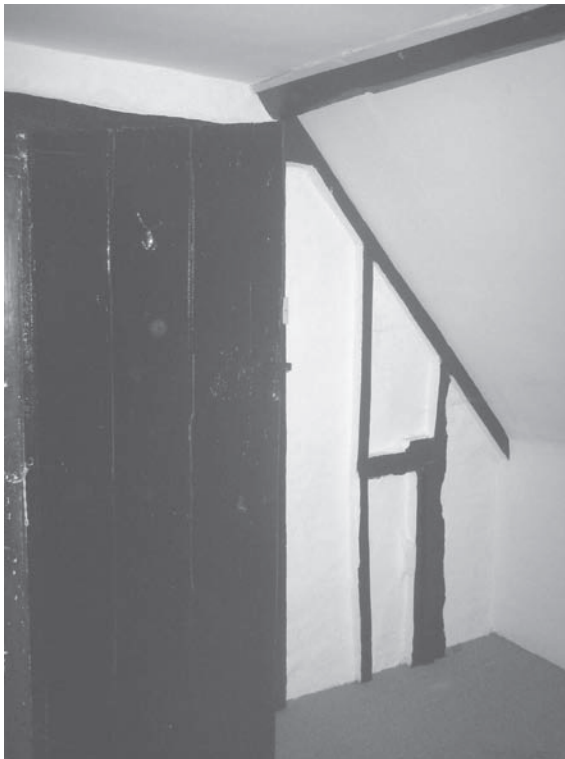
Fig. 5. The central truss. ( Photograph by David Clark. )
