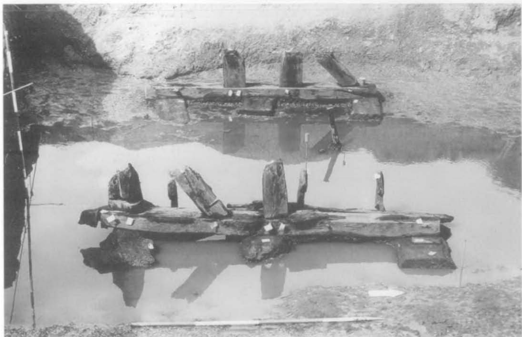
Fig. 2. Abingdon. Two trestles of a timber bridge dated by dendrochronology to c. 1510 AD, in the bottom of Convent Ditch (see Medieval Archaeology , xxxiv (1990), 206-7). (Photo: Oxford Archaeological Unit)
