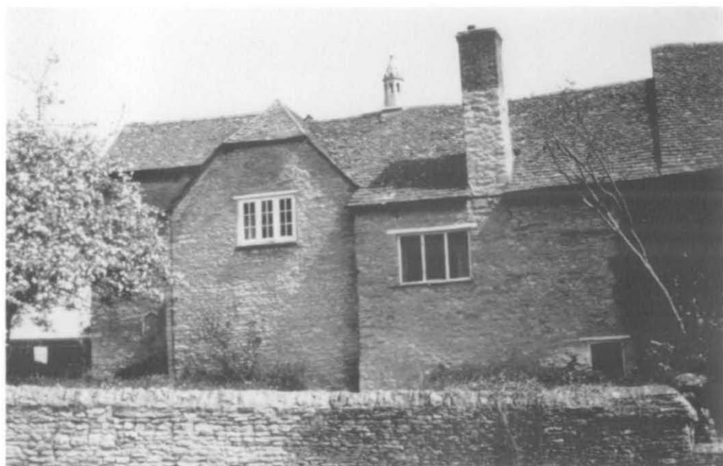
Fig. 1. The earlier range of Praunce's Place, viewed from S.W. Late 13th-century chamber-block in centre-right, with facsimile chimney-pot indicating the position of its original N.W. gable; late medieval 'tower' to far left.
