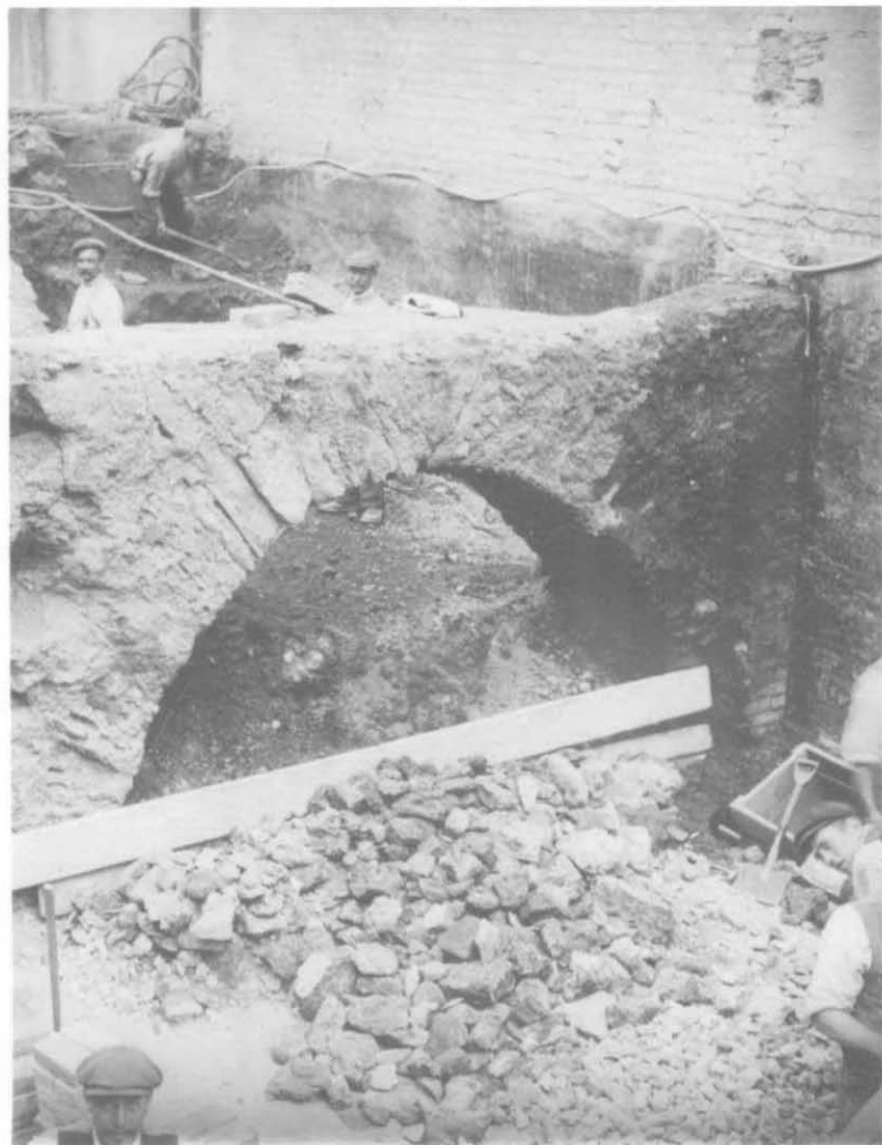
Fig. 19. Left : North range: view of relieving arch in foundation during demolition in 1911. Right : South range: view of west end during demolition in 1904, showing arch-braced roof. (Minn, Bodleian Library).
