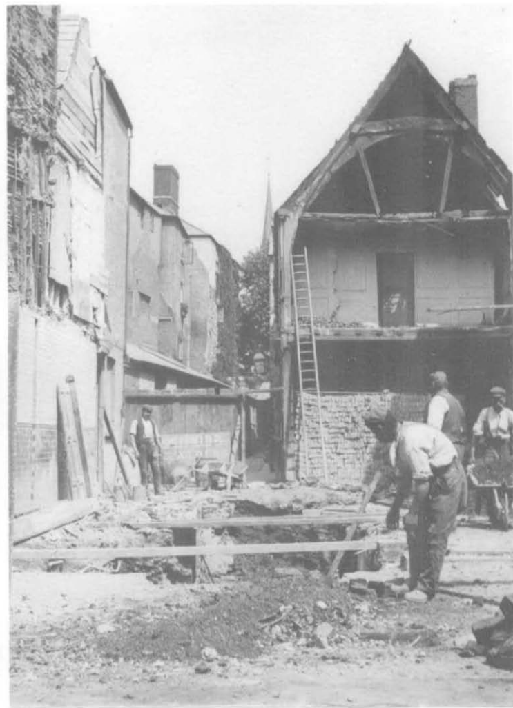
Fig. 19. Left : North range: view of relieving arch in foundation during demolition in 1911. Right : South range: view of west end during demolition in 1904, showing arch-braced roof. (Minn, Bodleian Library).
