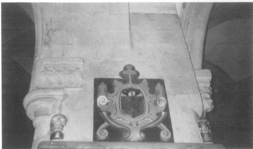
Fig. 62. Top of pier I.4 from the W., showing the thick transverse rib of the transept aisle vault, and the frieze of five-lobed leaves cut on the left by the 13th-century Lady Chapel work and on the right by the Goodwin monument. To the top-right is the undisturbed late 12th-century masonry of the S.W. corner of the pier. (Ph. John Blair.)
