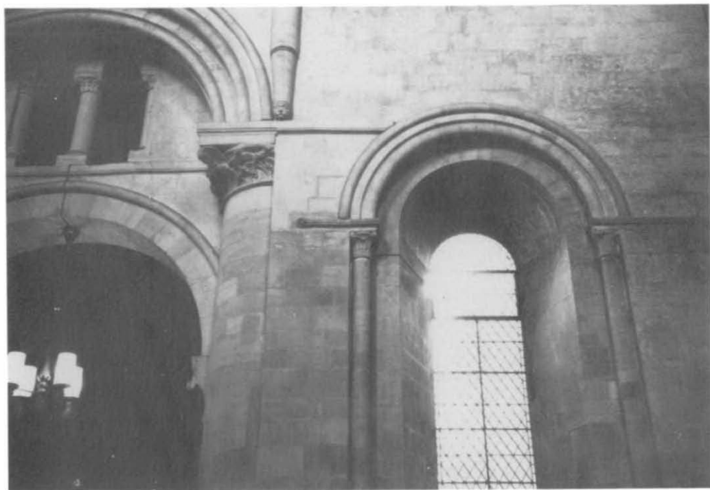
Fig. 56. Chancel N. side, to show awkward junction between abacus mouldings of arcade and window. (Ph. John Blair.)
