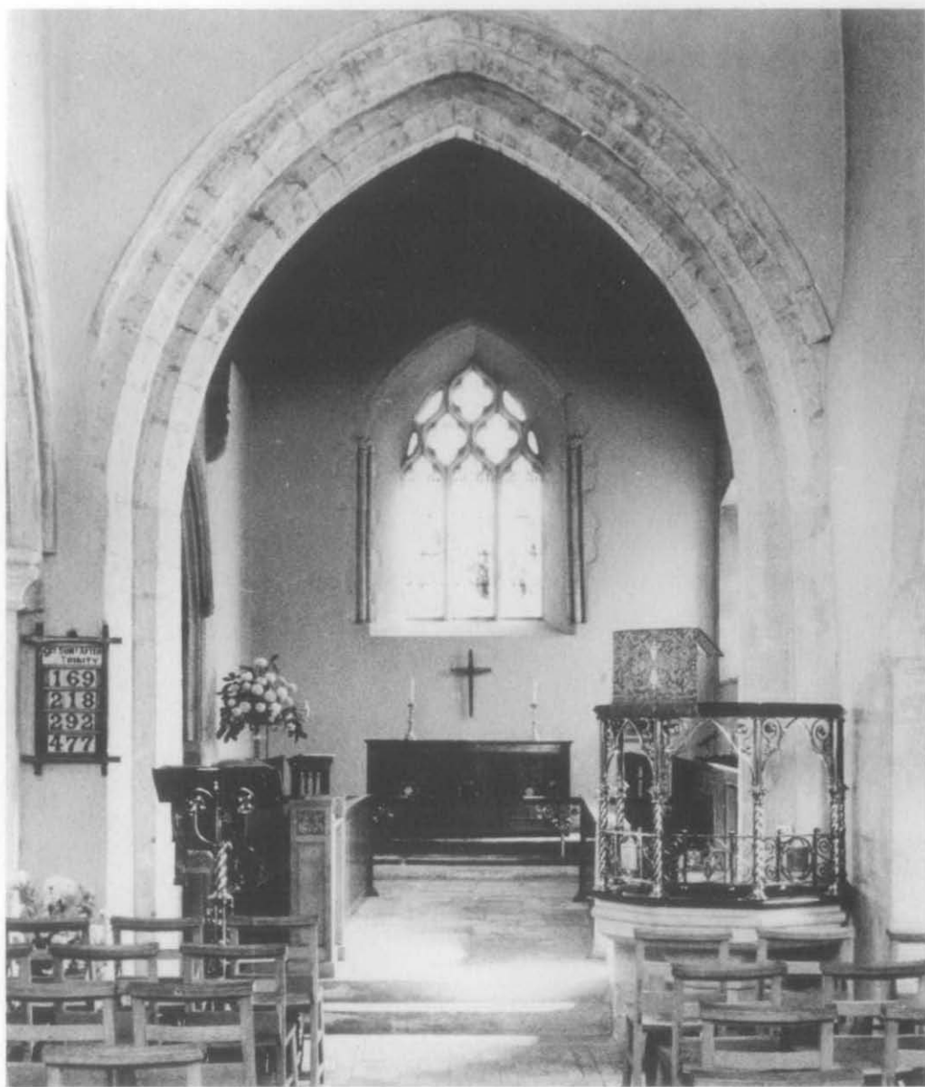
Plate 16. Cogges church: Interior looking east, showing Phase 3 chancel arch, and east window with Phase 3 rere-arch and shafts.
