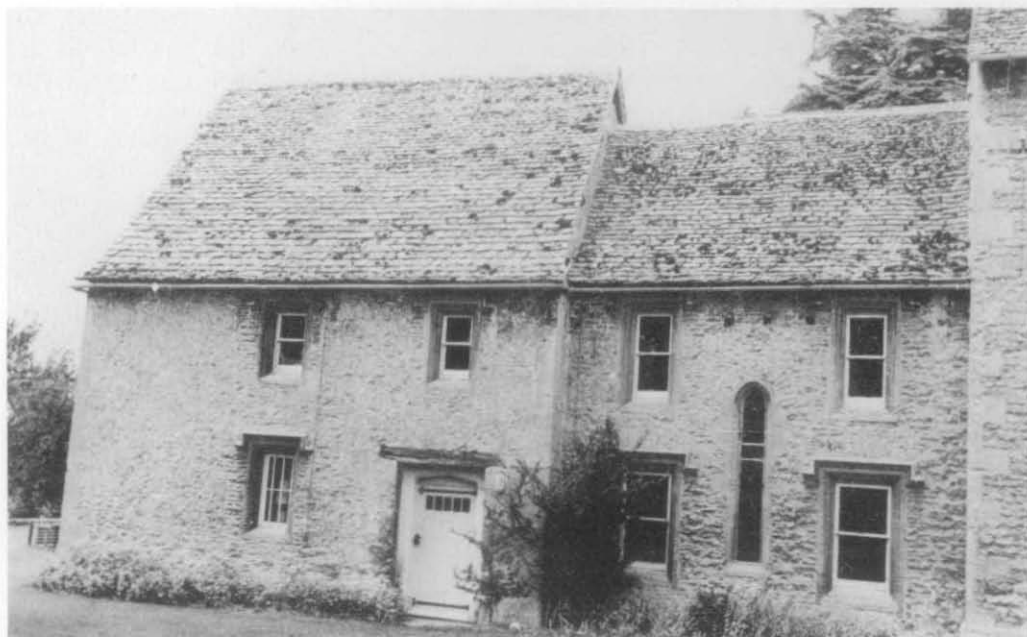
Plate 6. Cogges Priory: South-east elevation, showing (left) Phase 4 service-block as remodelled in Phase 5, (centre to right) Phase 4 hall, and (extreme right) corner of 1860 extension.
