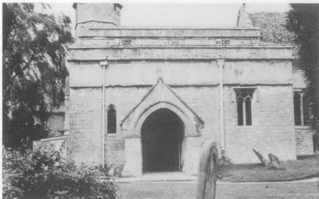
Plate 12. Cogges church: South elevation, showing Phase 2 south aisle (with later windows) and Phase 3 porch.
