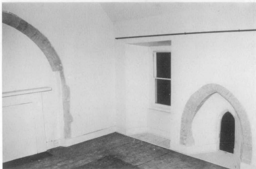
Plate 7. Cogges Priory: Upper room in Phase 4 hall, showing rere-arches of original windows.
