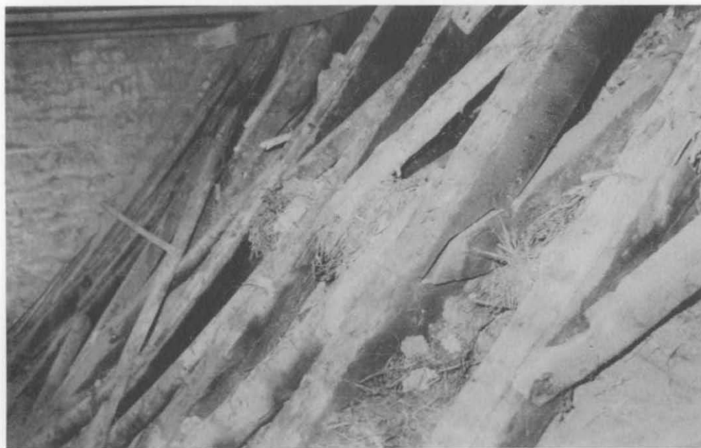
Plate 8. Cogges Priory: Exterior of original roof of Phase 4 hall, showing open notched-lap joints.
