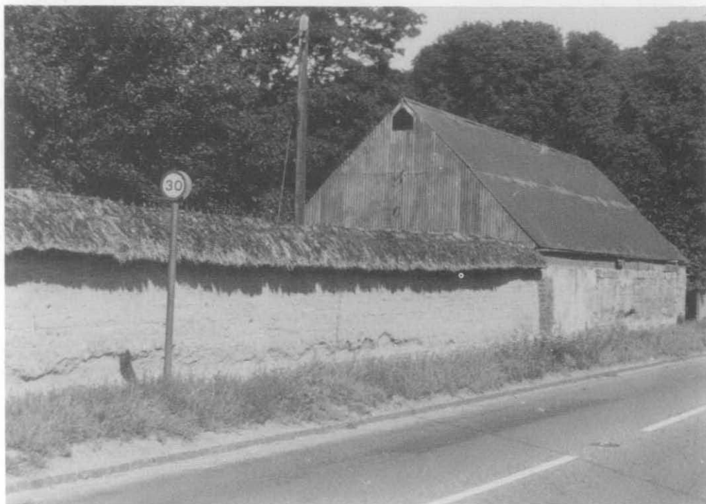
Plate 1. Thatched cob wall in modern Dorchester-on-Thames.
