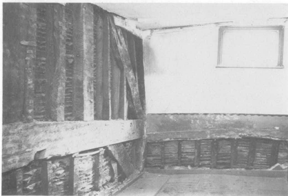
B. 24 New Inn Hall Street : first-floor room after plaster-stripping in 1975, showing the south face of truss A of the original building, and the top of the seven-barred window in the rear wall.
