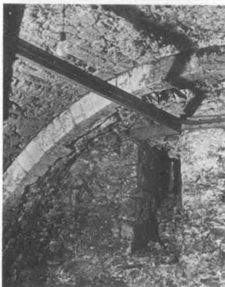
C. Frewin Hall subvault : part of westernmost arch, showing impressions of centring for vaulting.
