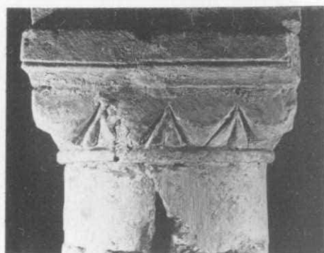
D. Frewin Hall subvault : capital of inserted column.
