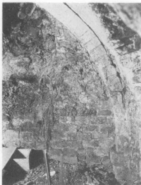
B. Frewin Hall subvault : part of westernmost arch, showing impost.
