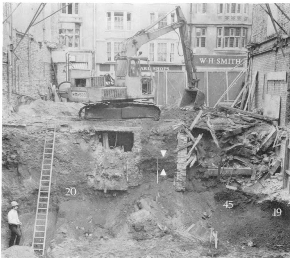
A. The middle of the site showing the existing basement and the depth of the excavation with pits 19, 20 and 45. Between the two arrows is an area of occupation resting on the brown loam which caps the natural gravel.
