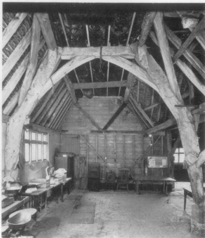
MIDDLE FARM, HARWELL. A, B. Cruck Barn. A, Exterior; B, North part of Truss III. C. Cruck Out-house, Open Truss.
