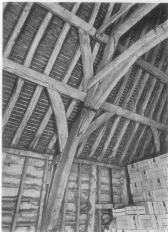
MIDDLE FARM, HARWELL. A, B. Cruck Barn. A, Exterior; B, North part of Truss III. C. Cruck Out-house, Open Truss.
