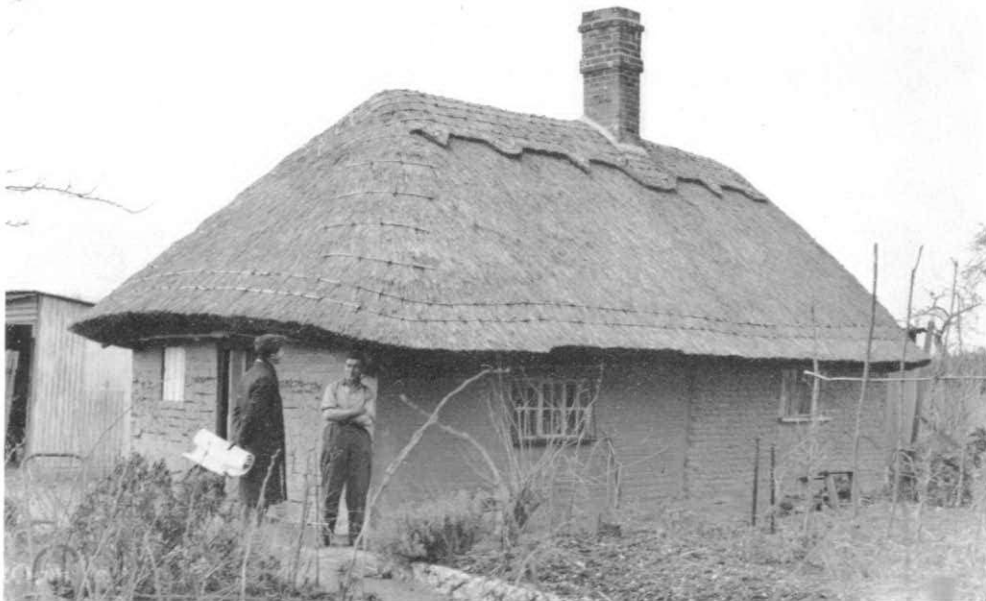
B. SQUATTER'S COTTAGE AT CHAZEY HEATH, JUST NORTH-WEST OF CAVERSHAM. THE WALLS WERE FORMERLY OF WATTLE AND DAUB BUT THE EXTERIOR IS NOW ENTIRELY OF BRICK
