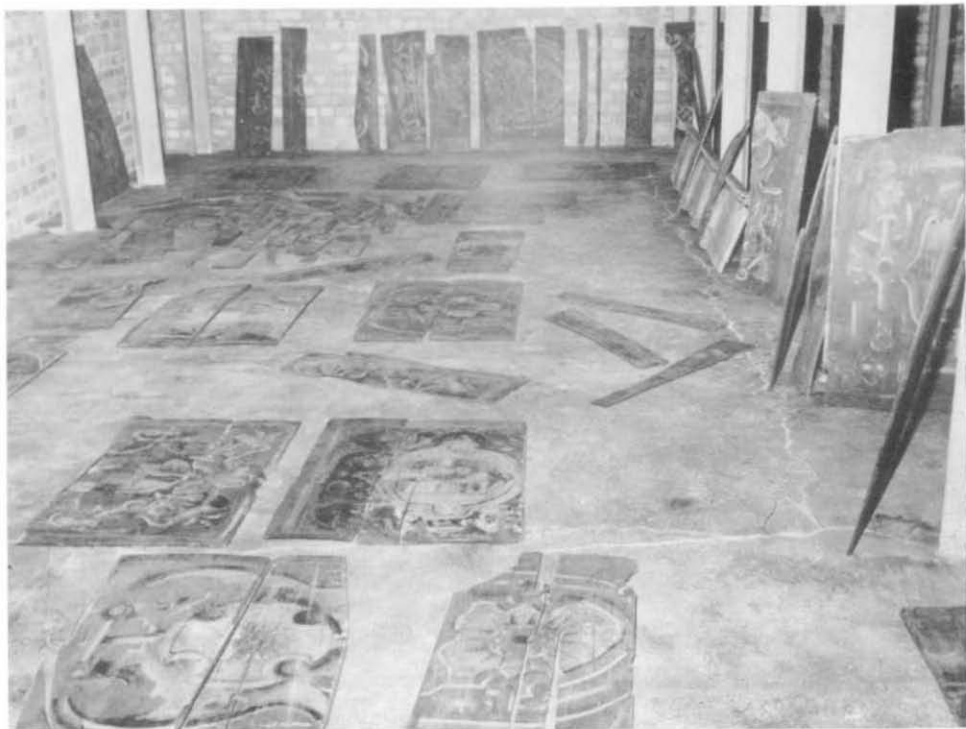
CHRIST CHURCH, OXFORD. Dismembered panels from the Old Library roof being re-assembled.
