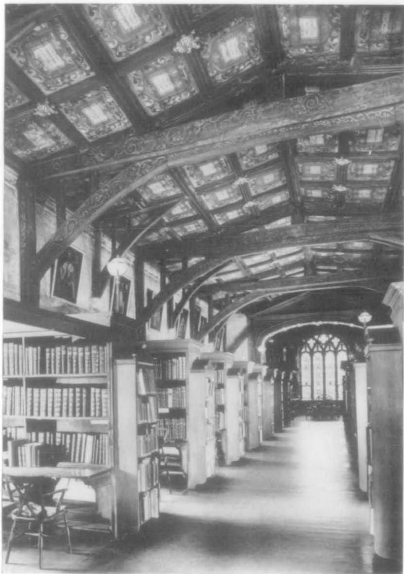
Duke Humfrey's Library, to show scroll-work on tie beams.
