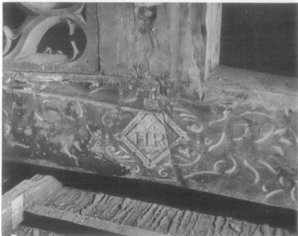
CHRIST CHURCH, OXFORD. The roof of the Old Library during dismantling. The device of Henry VIII. Note decayed area in 15th century beam boarded over and painted, c. 1610.
