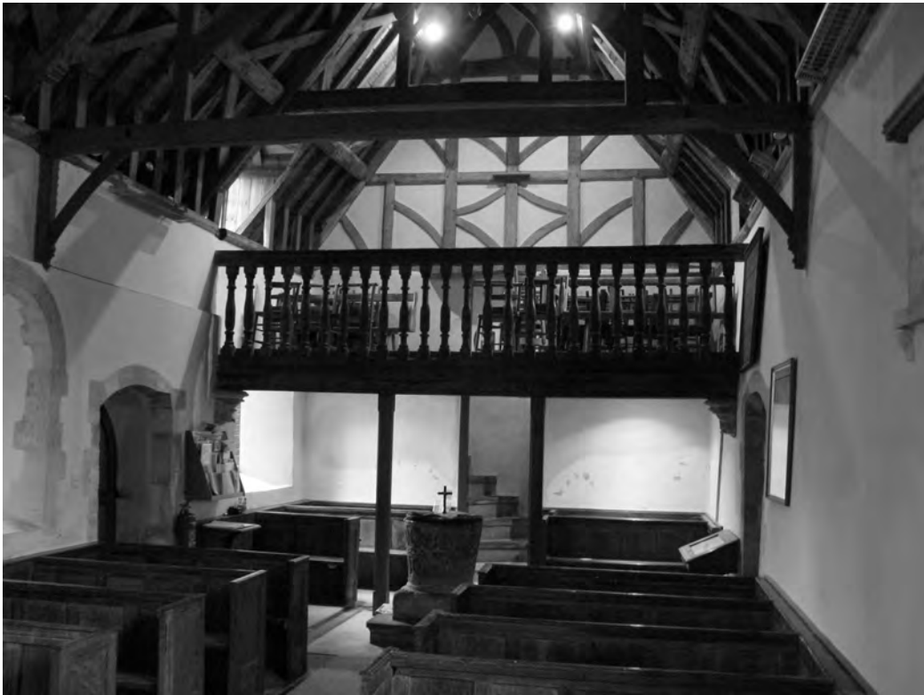
Fig. 6. Interior looking west, showing seventeenth-century roof and gallery, repositioned font and remodelled pews. Photograph by the author.
