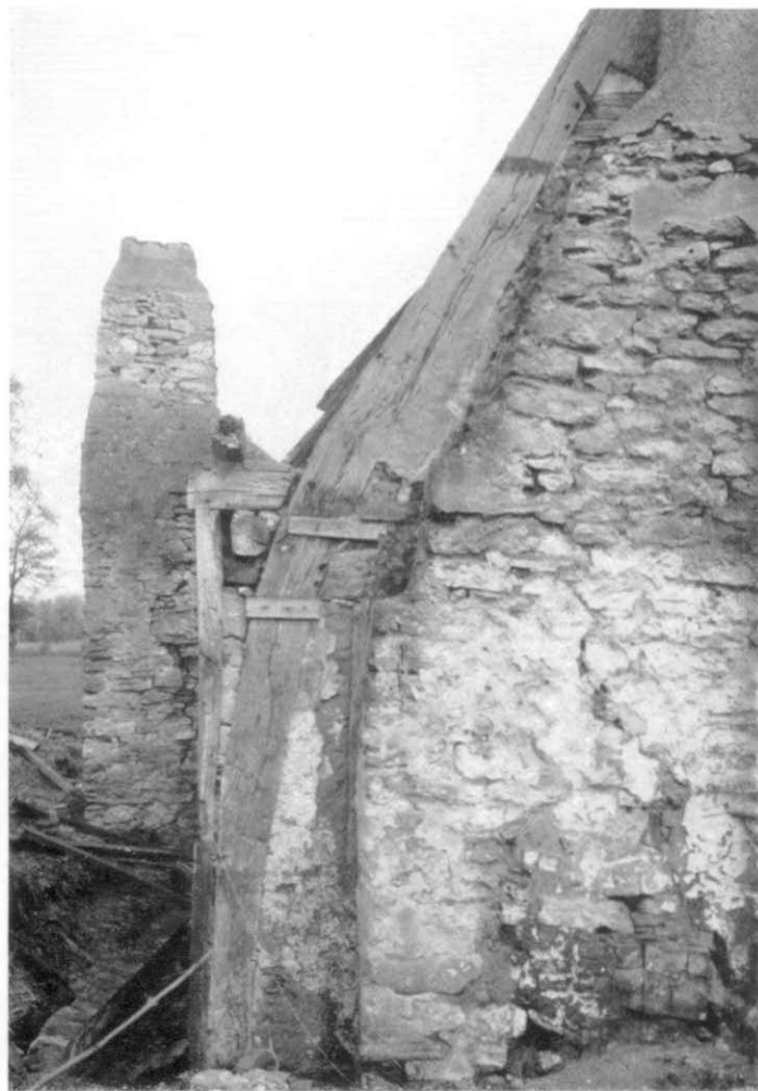
B. CRUCK I, NORTH BLADE FROM EXTERIOR
